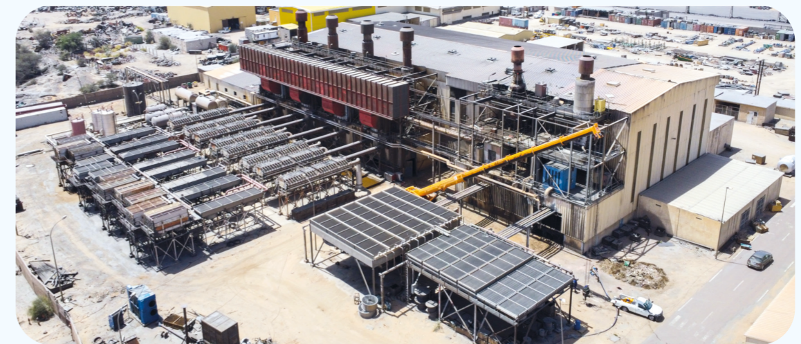
Zouerate thermal power plant station
