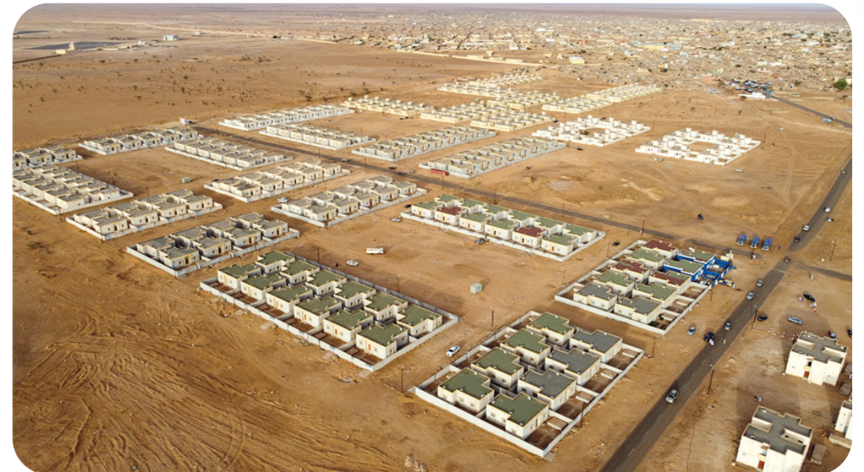
Part of the 600 housing units complex in Zouerate
